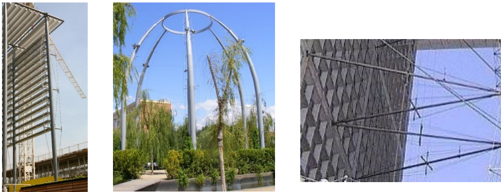
Fig. 1. Stayed members in Chiswick Park in London, Parc Central del Poblenou Barcelona, support of Grande Arche lift in Paris.
