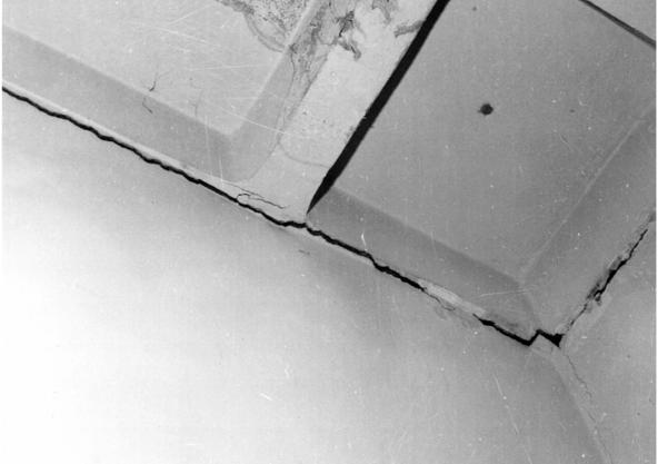
Separation of steel profile from a partition wall
