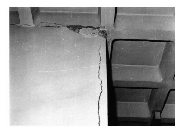
Department store in Prague cracks in a cladding wall nearby both ways cantilivered corner
