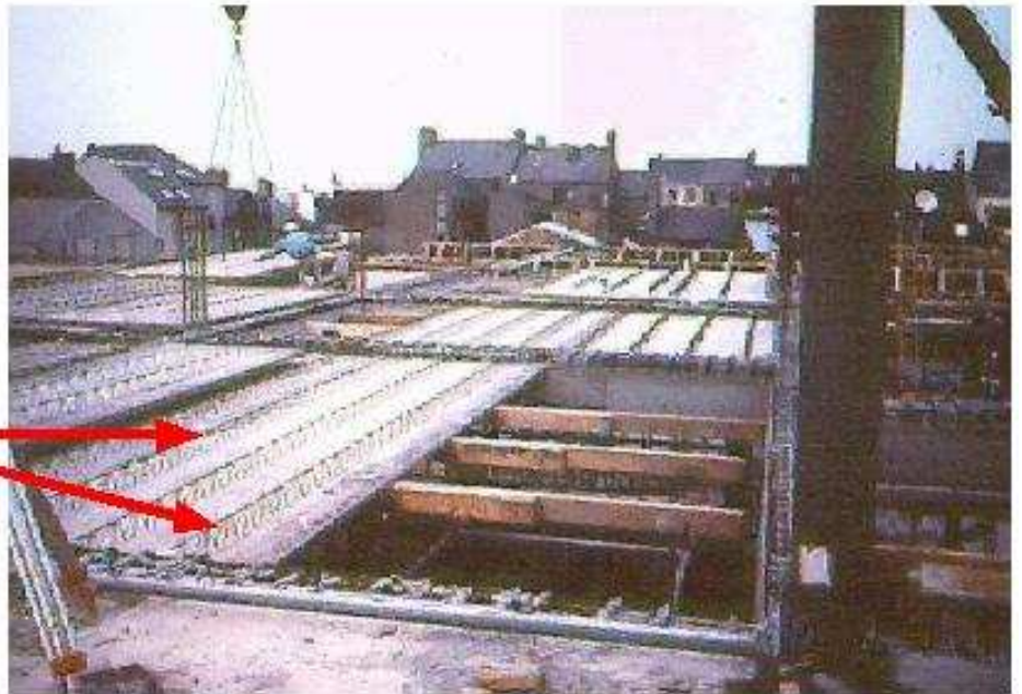
The triangulated lattice girders
