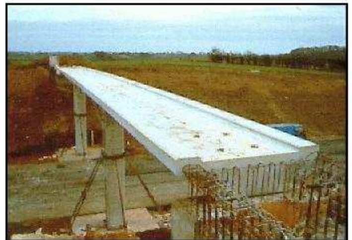
Long span bridge deck
