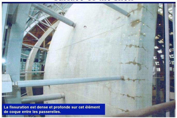
Rupture of concrete shell
